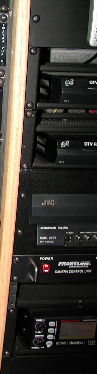
TWO VHF, UHF & 2 EACH 800 MHZ RADIOS ACU1000 BELOW RADIOS
